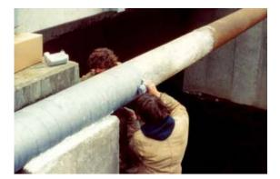
• Wax-Tape Wraps: microcrystalline waxes, plasticizers, corrosion inhibitors and other ingredients saturated into a nonwoven, nonstitch bonded synthetic fabric, forming a tape wrapper.
