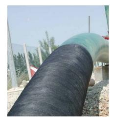
Rubber Outer Wraps: PVC film with synthetic rubber adhesives
