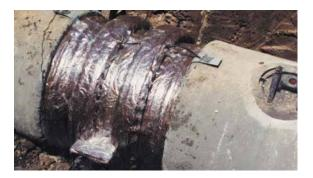
• **Polyester Outer Wraps:** spun bonded polyester mat saturated with microcrystalline wax that is laminated to a polyester film.
