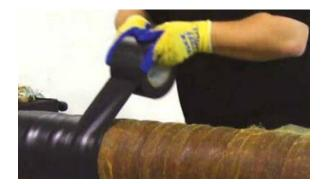
• **Plastic Outer Wraps:** three membranes of clear, polyvinylidene chloride high cling- plastic wound together as a single sheet.
