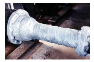
• **Curing Outer Wraps:** specialized blend of quick-curing resins impregnated into a polyester fabric.
