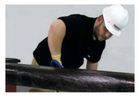
• Wax Tape Primers: blend of microcrystalline waxes, plasticizers, and corrosion inhibitors. Have a paste-like consistency and designed to displace moisture and wet the surface ensuring adhesion of the tape.
