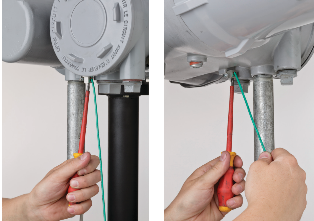
Figure 3-5 Earth/Ground Connection
