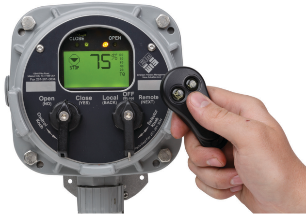
Figure 4-1 TEC2 Controller
