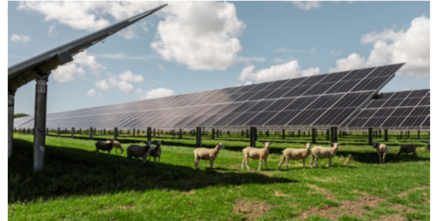
Lodestone is the first first company in Aotearoa to adopt agri-voltaic technology that allows livestock to graze around the solar arrays.
