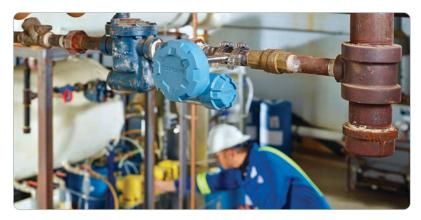
When paired with Emerson Plantweb Insight applications, the non-intrusive Rosemount 708 Wireless Acoustic Transmitter can help to diagnose faulty steam traps and pressure relief valves that contribute to greenhouse gas emissions.
