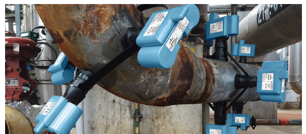
Emerson's Rosemount Wireless Corrosion and Erosion Transmitters continually monitor for both corrosion and erosion.
