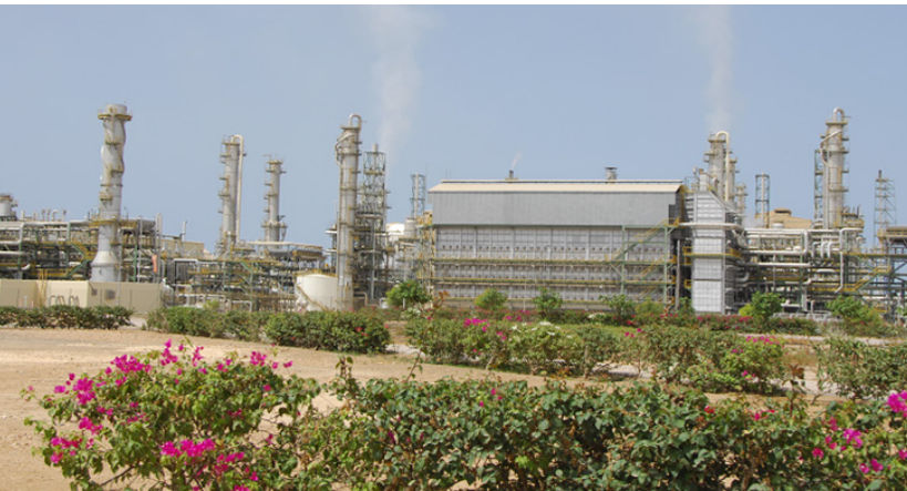
With high demand for its products, ensuring smooth operation of critical equipment is a top priority for OMIFCO
