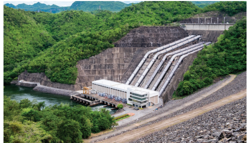
Figure 5.13: Flow measurement through long distance municipal water gathering lines pose the dual challenges of large size and remote site conditions.
