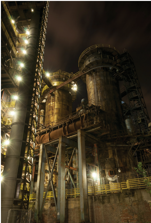
Figure 5.3: A blast furnace, where cooling systems should be monitored for proper flow to prevent damage or hazardous conditions.
