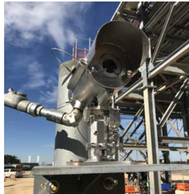
Figure 14: Fixed point combustible and toxic gas detectors use multiple sensor technologies, such as infrared, catalytic bead and electrochemical. The Rosemount 925FGD Fixed Gas Detector (left) can detect all flammable gases and common toxic gases. Rosemount 935/936 Open Path Combustible and Toxic Gas Detectors (right) use infrared and ultraviolet technology to detect hydrocarbon and toxic gases, including methane, propane, ethylene, hydrogen sulfide and ammonia.
