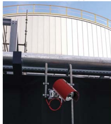
Figure 15: Rosemount 975 Multi-Spectrum Ultraviolet & Infrared Flame Detectors respond to the specific wavelengths of light produced by a variety of burning fuels.
