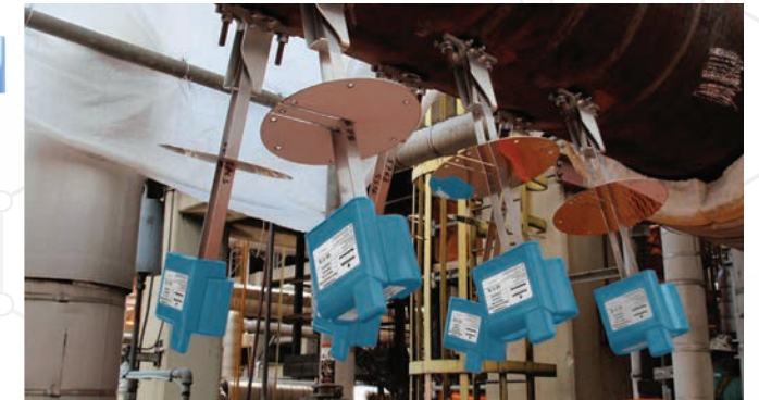
Figure 17: Rosemount Wireless Permasense Corrosion and Erosion Monitoring Systems measure wall thickness continuously so maintenance can determine when pipe must be replaced.
