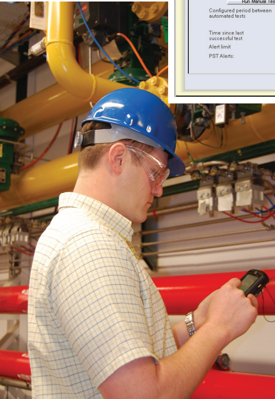
← Figure 3. For safety reasons, an operator must start the partial-proof test, either locally or remotely.
