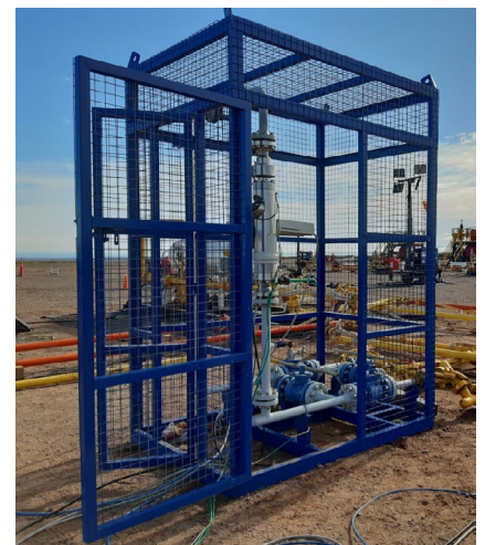
Image 1. The Roxar 2600 MPFM installed on site during trial testing
