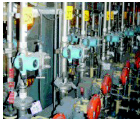
Rosemount 3051SFP Integral Orifice Flow Meter pipe rack skid with the "drop-in" solution
