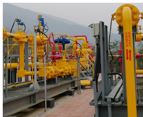
Bottom: Customer's LNG skid with Rosemount 3051S MultiVariable Transmitters and Rosemount 585 Annubar
