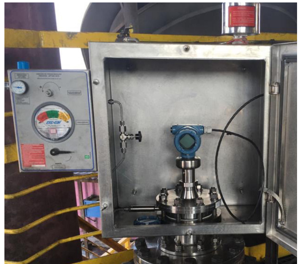
Rosemount 5408 mounted inside a cooling box
