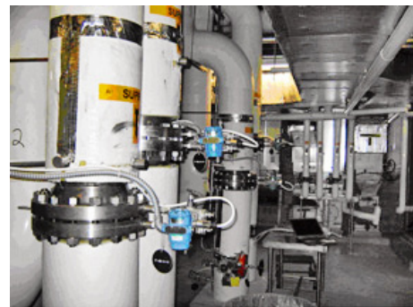
Conditioning Orifice Mass Flow Meter (1595 Conditioning Orifice Plate with MultiVariable Transmitter)
