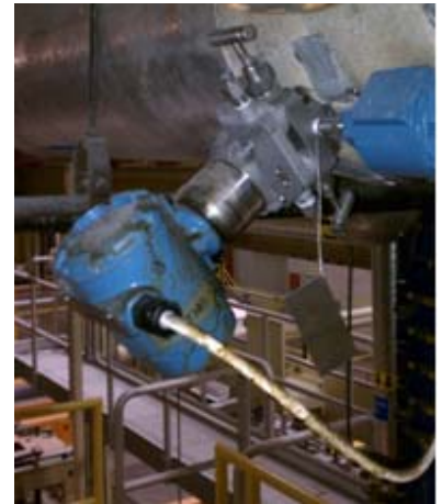
Rosemount Compact Annubar Flow Meter installed between two raised face flanges.
