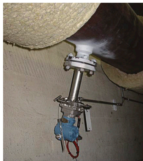
Installation of the Rosemount Annubar Flow Meter
