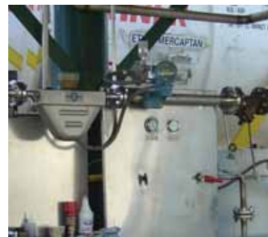
A corporate SAP system calculates inventory levels based on Micro Motion mass flow custody transfer measurements for incoming raw materials and out-going products.
