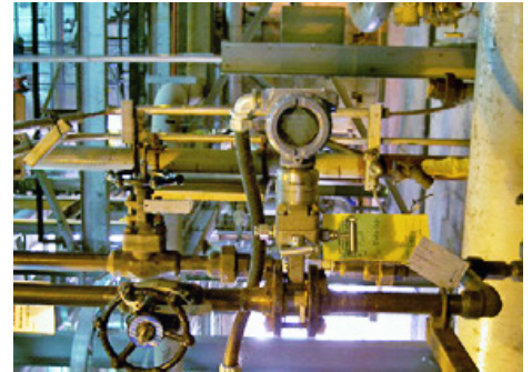
Rosemount 3051S Differential Pressure Transmitter with 405P Compact Orifice
