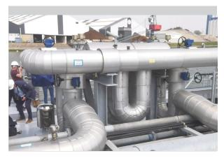
NMI-certified metering system based on Emerson's Micro Motion High Capacity mass flow meters loading up to 3000 tonnage/hour of fuel oil, used onboard Vorstenbosch, the biggest bunker barge in Europe
