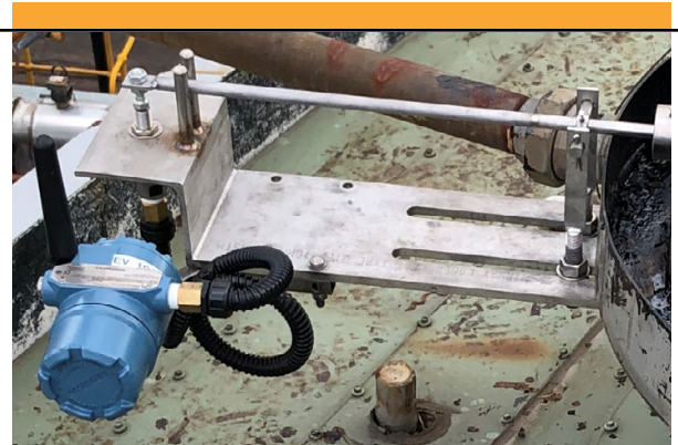
An in-house designed mechanical movement amplifier that enables minute vent lifts to be detected by the Emerson GO Switch and Rosemount 702 Wireless Discrete Transmitter.
