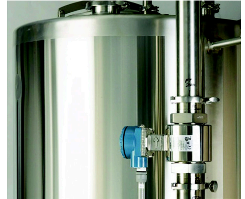
Rosemount 8721 Hygienic Magmeter installation
