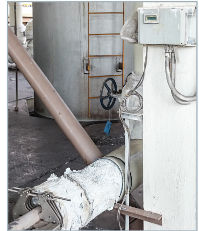
Measuring point with WaveInjector® and FLUXUS® F704 A2 transmitter
