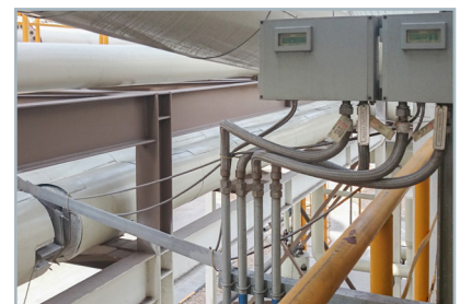
Measuring point with WaveInjector® integrated into the insulation
