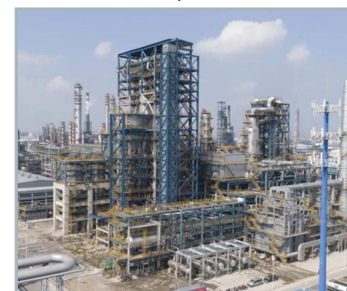
The Sinopec ZRCC hydrocracker under construction
