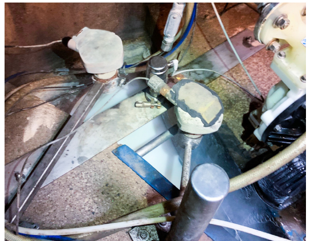
The Rosemount 1408A is installed in a parshall flume, next to old legacy devices.
