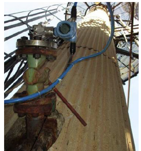
Rosemount™ 3051ERS installation
