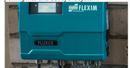
The FLUXUS® F721 TE is used as the measuring transmitter for stationary heat quantity measurements.
