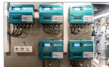
Energy measurement systems of the type FLUXUS® F721 TE in dual channel design are mainly used.
