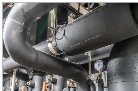
Measuring point for thermal energy on a cooling line. The ultrasonic and Pt100 temperature sensors are fully integrated into the insulation.
