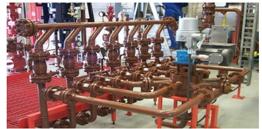
Image 3. Manifold and Fisher Multiport Flow Selector (MPFS)
