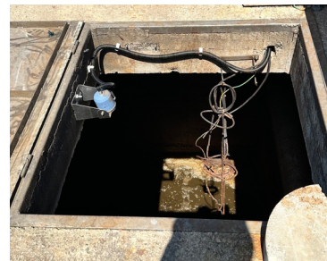
Image 2. The Rosemount 1208 uses radar technology and is unaffected by process or environmental conditions.
