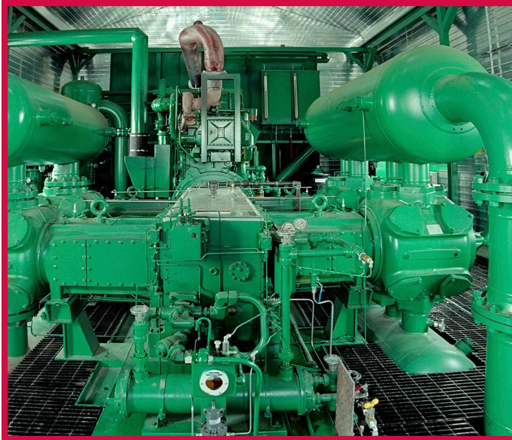
For 90% of the malfunctions, vibration, temperature, and process measurements can be monitored to detect changing conditions early, so you can avoid an unplanned shutdown. A basic monitoring program on reciprocating compressors can save you 30% or more in unplanned downtime and keep man and machine safer.
