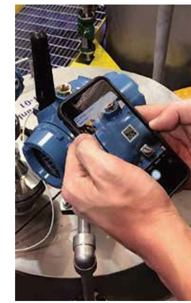
Scan the QR code on the device for serialized device information in the field.
