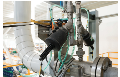
Emerson's pigging technology enables the efficient transfer of several products through a single line without cross-contamination.
