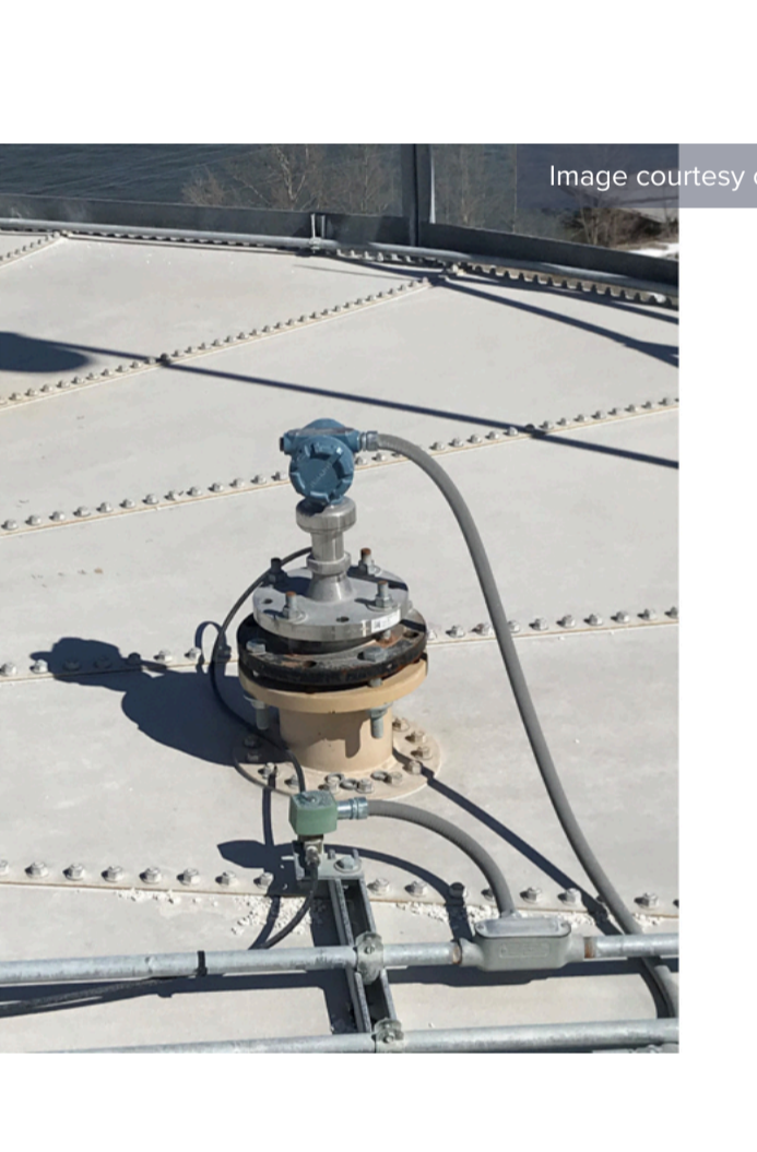
Figure 4: The Rosemount 5408 non-contacting radar provides robust measurements without the need for regular cleaning.
