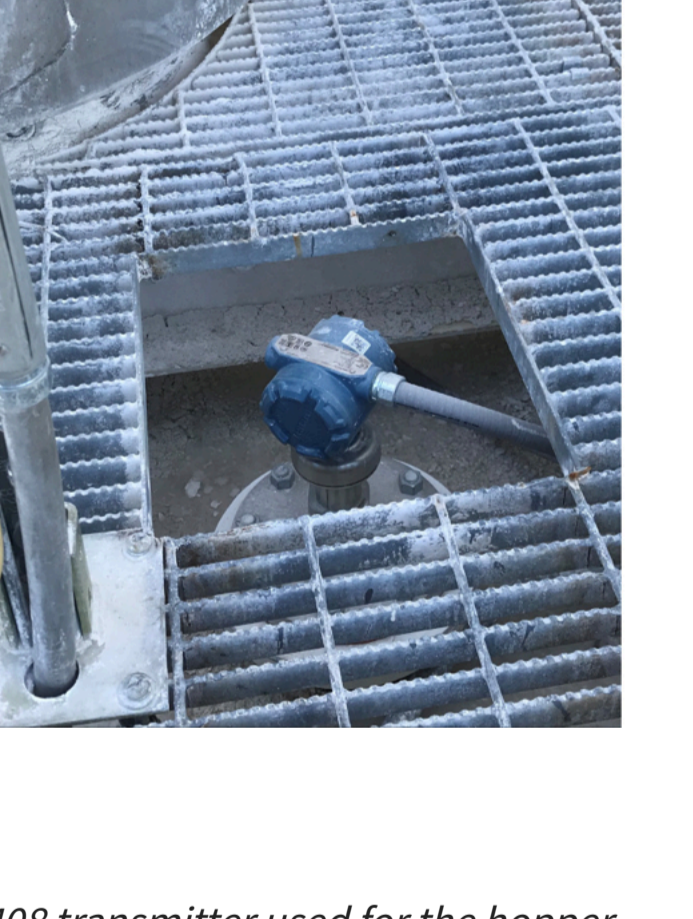
Figure 6: The Rosemount 5408 transmitter used for the hopper.
