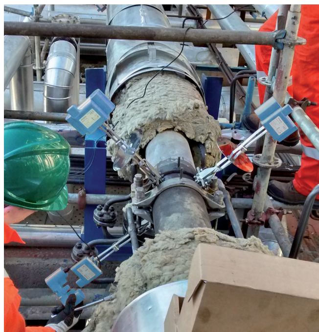
Figure 6 Example installation of Rosemount WT210 Transmitters
