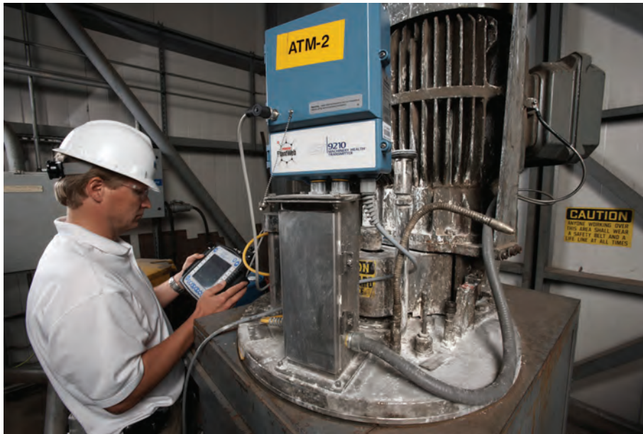
Figure 4 - Checking Vibration Readings at Atomizer 2.
