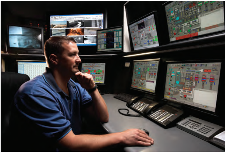
Figure 2 - Keeping tabs on the equipment's condition from the control room at Elk River Station.
