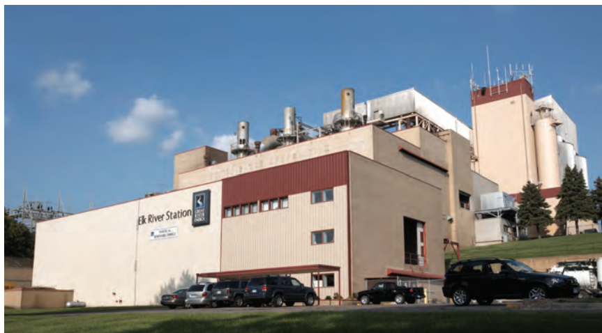
Figure 1 - The Elk River Station is a Waste-to-Energy facility, which creates enough electricity to power about 30,000 homes.
