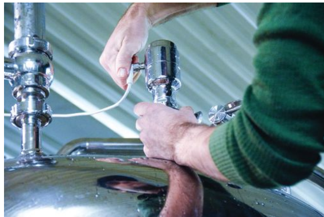
◀ Installing the Rosemount 1408H non-contacting radar level transmitters on the fermentation tanks was straightforward and they proved easy to use, which was crucial for the brewery.
