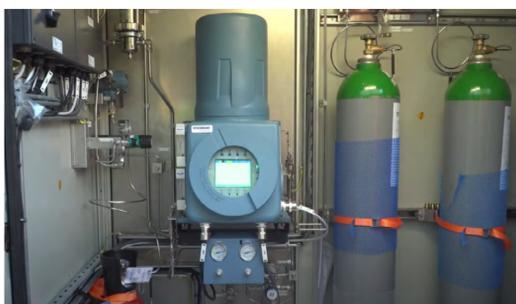
Green hydrogen producer ensures the quality of the network's gas blend using a gas chromatograph.
