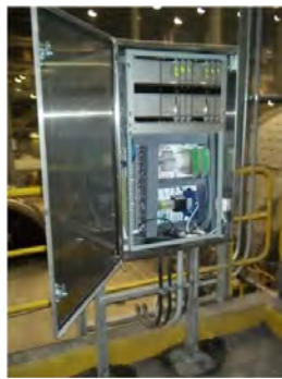
Figure 4-5: A6500MR in a full wall-mount enclosure (48 channels shown)
