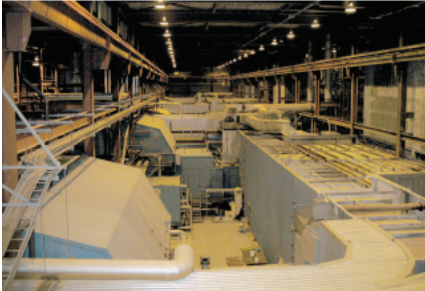
3. Gas turbines as they look leaning over the turbine-deck rail. The heat-recovery steam generator serving the first GT in the picture is to the right
