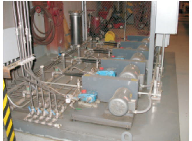
11, 12. On a hot, dry day fogging can boost engine output by about 5 MW. Both Caldwell (left) and Mee systems (right) serve Stony Brook
