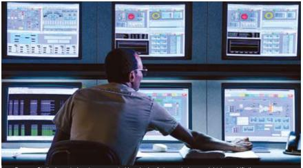
Pawnee Station's control system generated hundreds of alarms during an eight-hour shift; there were 39,000 possible alarm configurations. Photo courtesy Xcel Energy.
